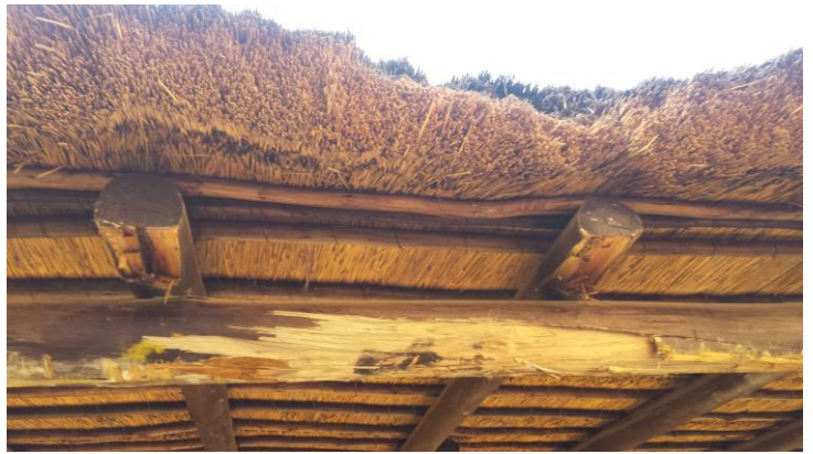
June 2017 - Damaged roof of Nature Reserve entrance
