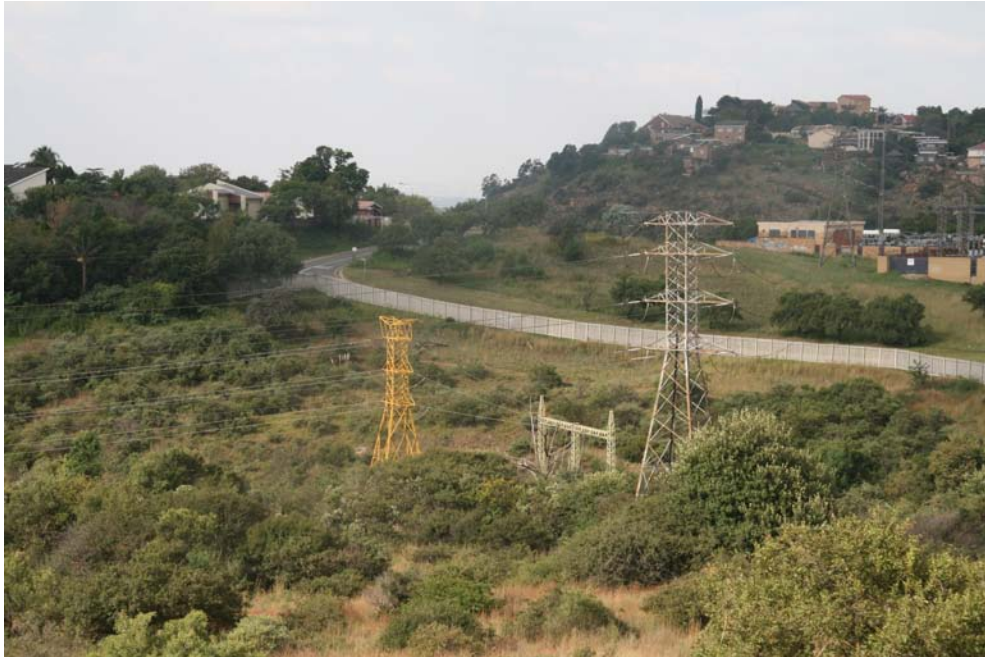
Figure 10. Powerlines cross the KDNR and markers should be installed to prevent bird collisions with the lines.
