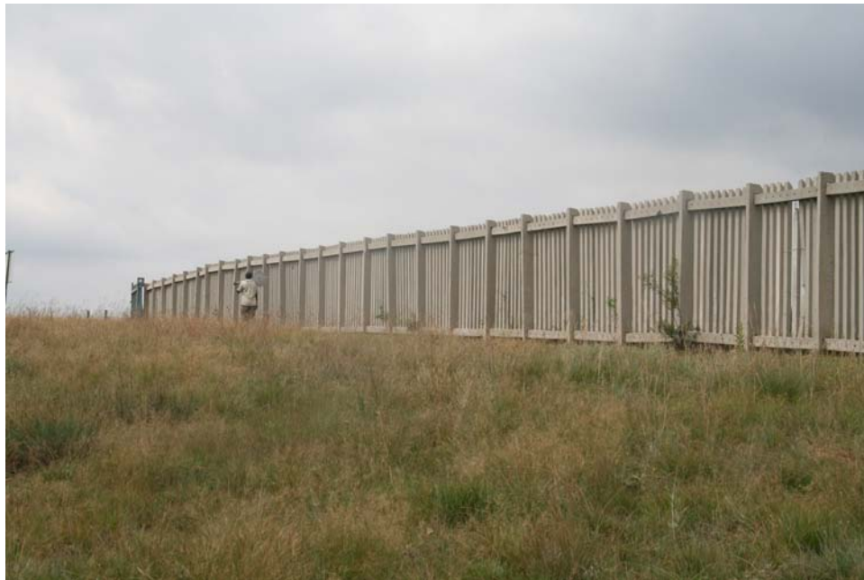
Figure 1. Most of the perimeter of Kloofendal Nature Reserve is fenced with a concrete fence.
