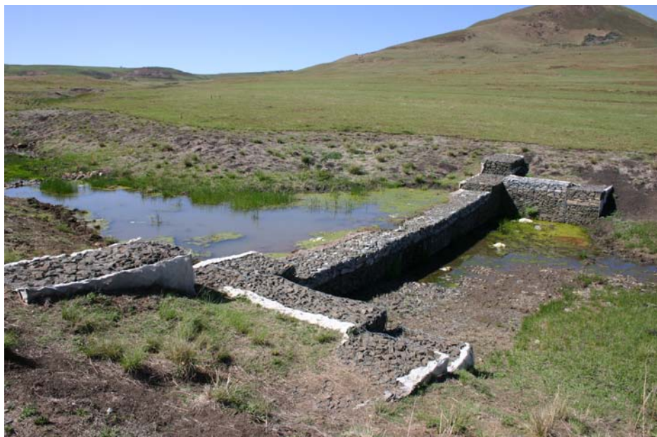
Figure 13. Example of gabion structure to control erosion and stabilize drainage lines or provide water for animals.
